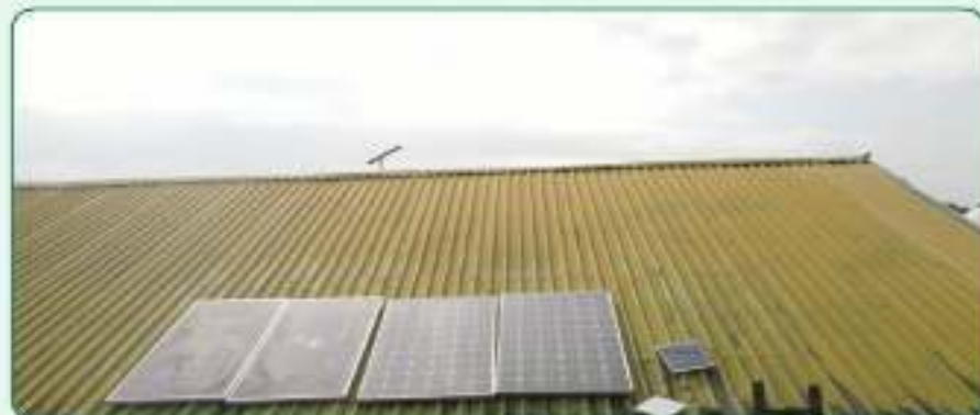
Solar panels & Starlink on the health center roof
